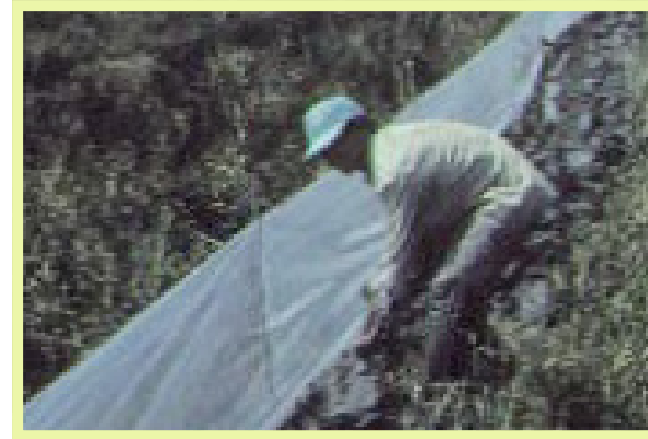
Figure 44: installing the plastic fence of a Trap Barrier System with the cage inside at the fence; this TBS now awaits planting of traps crop and construction of moat around the outside perimeter.
