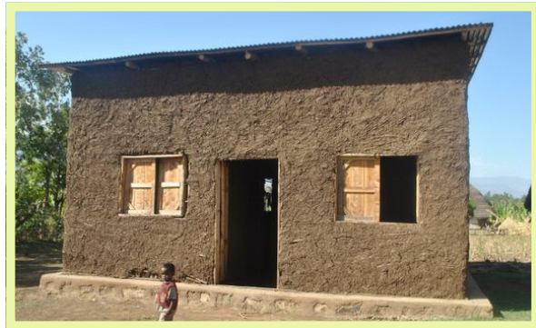
Figure 14: example of clean houses with concrete at the bottom part to prevent rats to enter
