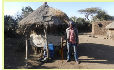
Figure 19: A farmer standing next to an outside grain store made from wood walls painted with dung and covered with grassed roof. The floor of the store is about half a meter hanging above the ground (borrowed from Meheretu et al. 2019).
