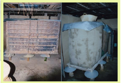
Figure 16: A barn in the house painted with cow dung which made from bamboo and wood and has round barriers on the legs/posts to control rat from climbing
