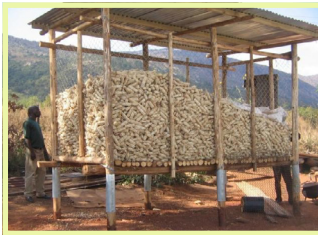
Figure 17: Good storage structure raised on poles
