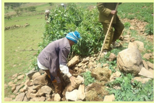
Figure 35: bad example: low quality stone bunds invite rats to take shelter
