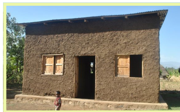
Figure 14: example of clean houses with concrete at the bottom part to prevent rats to enter
