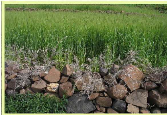
Figure 37: make the other stone bunds at sufficient distance from each other
