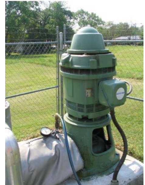
Well with electrically powered pump
