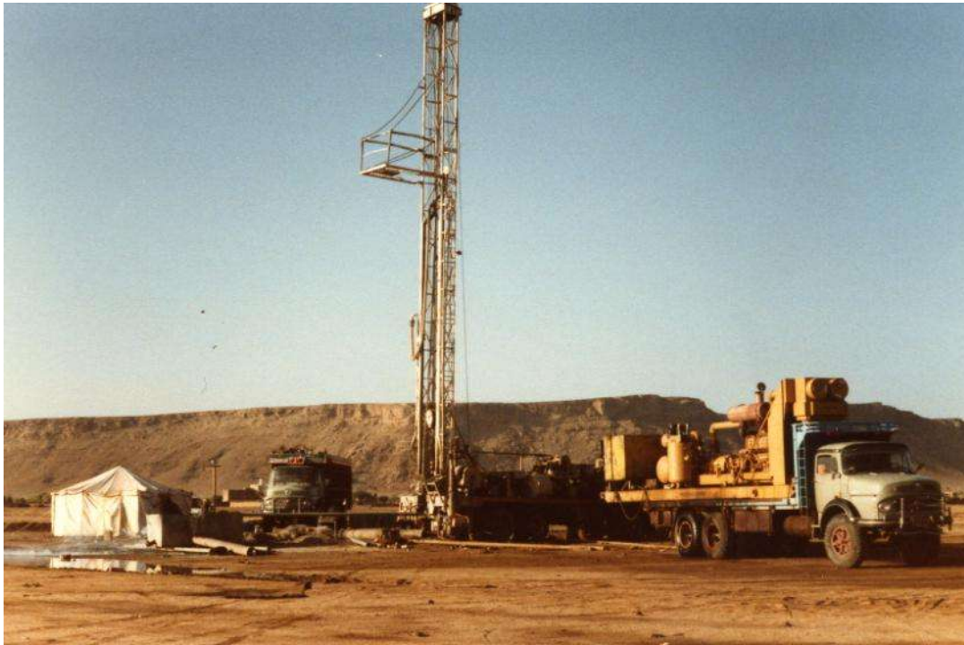
Drilling a well
