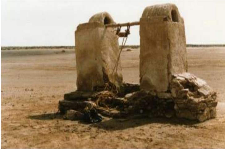
Dug well with pulley, rope and bag
