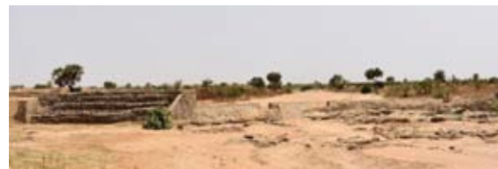
Figure 21. View from downstream of the dam
