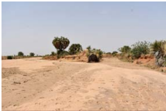
Figure 18. Diversion canal upstream Baba dam
