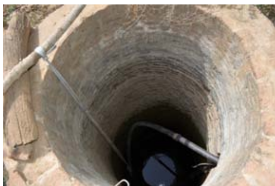
Figure 22. Water available in wells due to recharge from the dam
