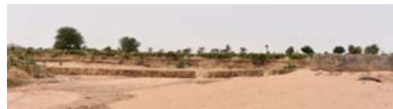
Figure 20. View from upstream of the dam
