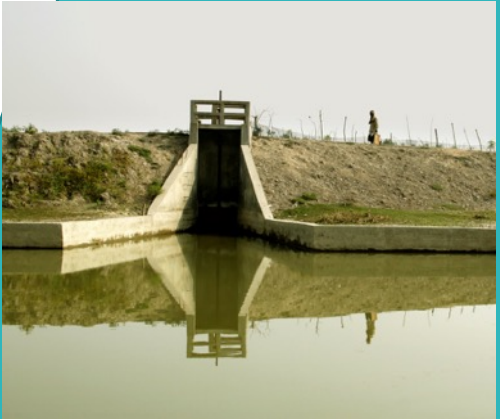
Water infrastructure rehabilitation
