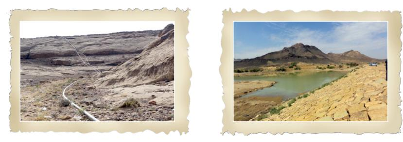
Farmers in wadi Areesha, Sana'a Basin, come together with support from the government to construct a dam for groundwater recharge. Well drilling is allowed around the reservoir area and water is pumped to the farms upto 4 km distance
