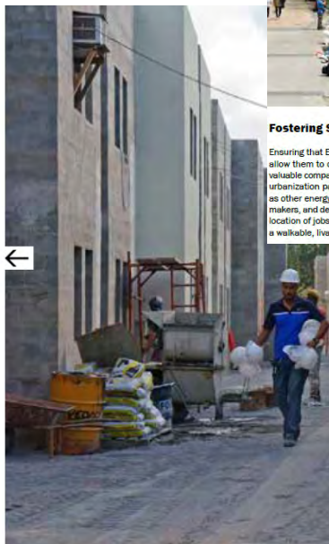
Masons work at a new condominium at Sao Bartolomeu, a low-income neighborhood in Salvador, Bahia. Hundreds of families who were constantly exposed to floodings and landslides will be relocated to the new buildings. Source: Mariana Ceratti / World Bank, CC BY 2.0, https://creativecommons.org/licenses/by/2.0/legalcode
