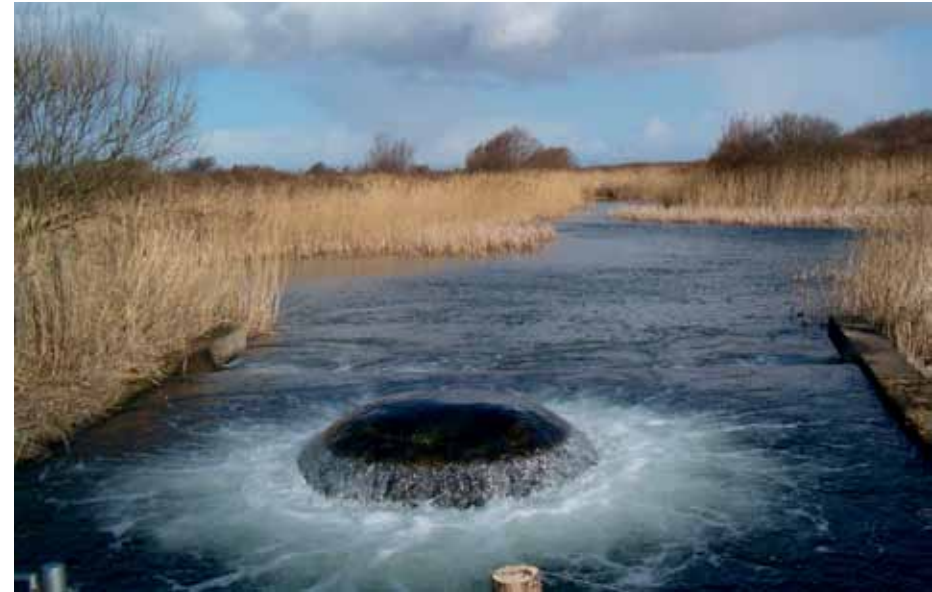
Photo 5. River water infiltration in sand dunes for drinking water, The Netherlands.
