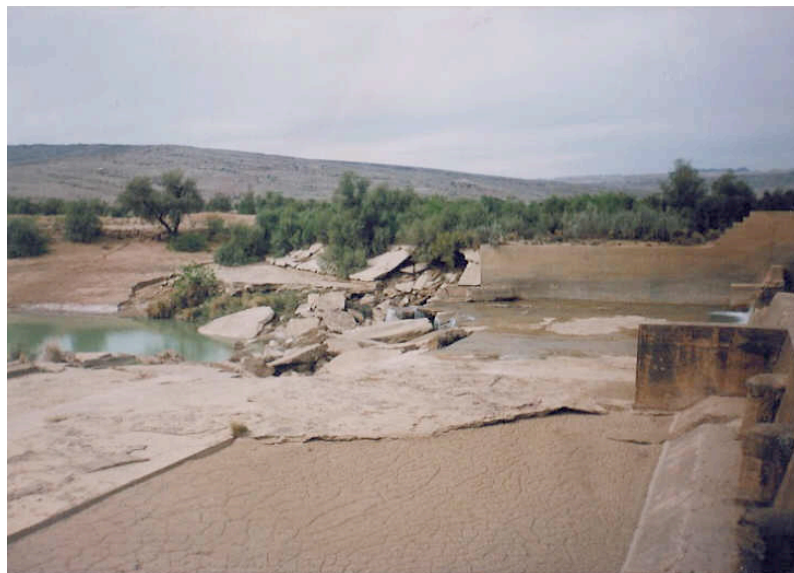
Figure 6 Diversion weir where part of the crest was blown by farmers as it interfered with the base flows, Pakistan
