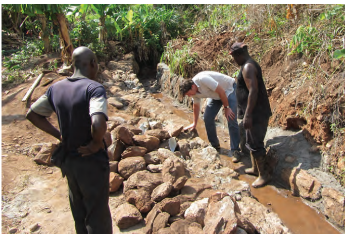
Picture 14: Involving local artisans in construction to build local capacities (Credit: Gert Jan Veldwisch)
