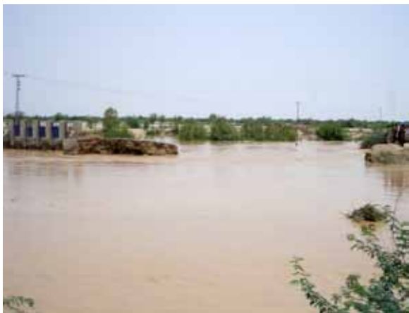
14.2 Damage after 2010 massive floods
