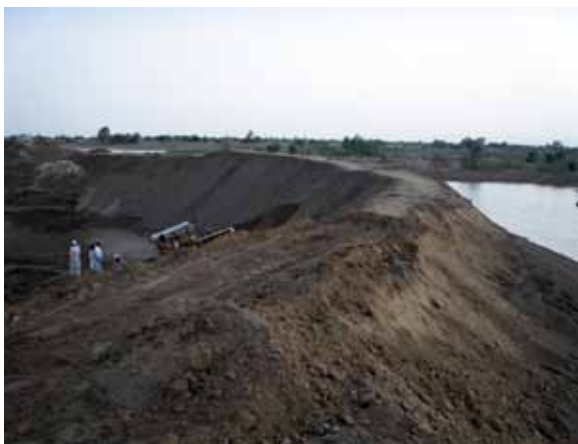
2.2 Repair of diversion bund D.I. Khan
