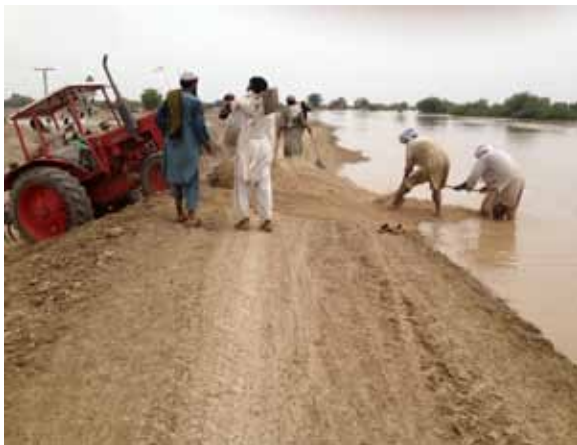
10.1 Plugging seepage hole in guide bund
