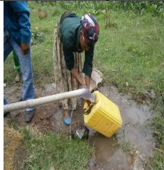
Large diameter outlet pipe so pipe does not fit into the jerrycans. Suggestion to reduce diameter outlet pipe to 1 1/4"
