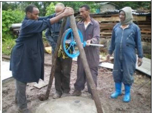
Installing pole model pump
