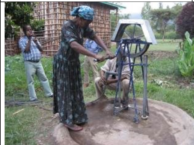
Pump connected with a hose for garden irrigation
