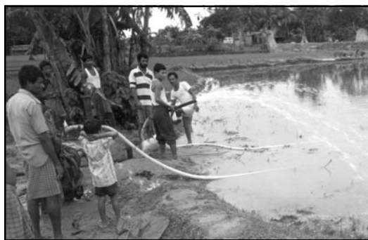
Figure 10 Jetting tool, using horizontal jets
