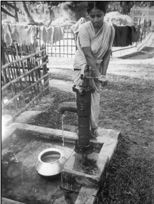
Figure 1 Hand pump, used for drinking water and vegetable irrigation
