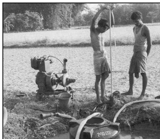
Figure 12 A well being washed with a surge piston
