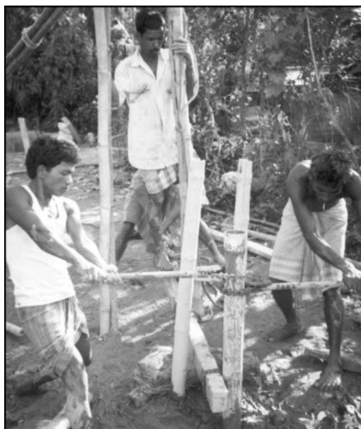
Figure 3 Back and forth movement of pipes
