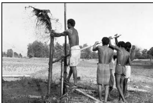
Figure 3 Drilling in progress for a shallow tube well
