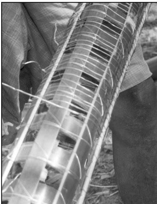
Figure 5 An iron rod frame
