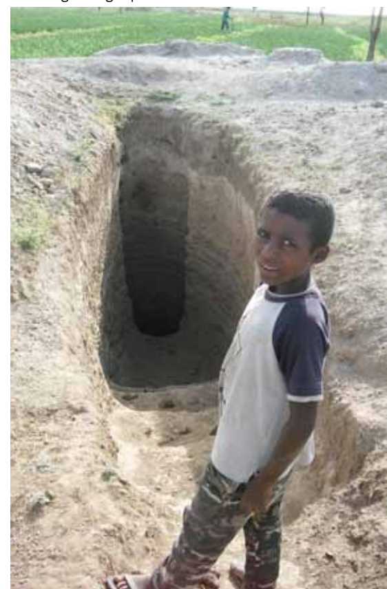
Figure 2: Dugwells in flood plains: prone to collapse and vulnerable to lowered water tables (Photo credit: MetaMeta)
