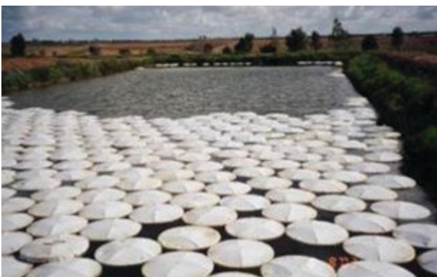
Photo 5: Example of Aqua Caps (Source: Youssef, Y. W., & Khodzinskaya, A. (2019). A review of evaporation reduction methods from water surfaces. In E3S web of conferences (Vol. 97, p. 05044). EDP Sciences.)
