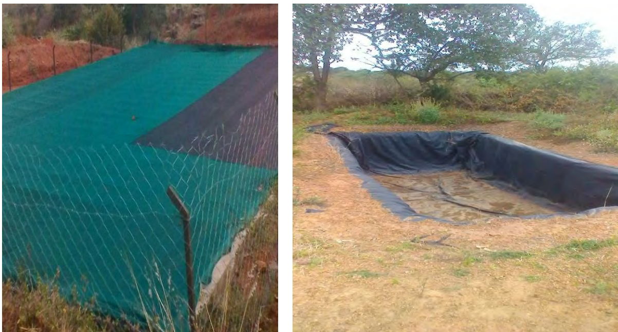
Figure 8 examples of ponds to store surface/road harvested water
