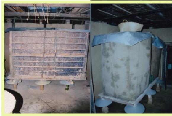
Figure 19: Barns in the house; on the left made from wood and metal, on the right made from wood and bamboo, painted with cow dung. See again the round disks on the poles, these prevent rats from climbing up.
