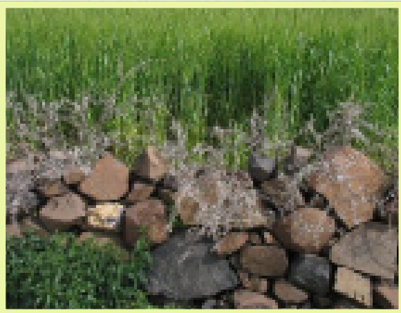
Figure 40: Make the other stone bunds at sufficient distance from each other
