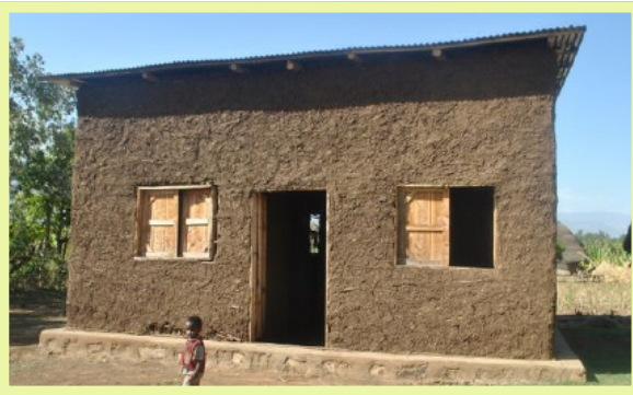
Figure 14: Examples of clean household compounds and houses with concrete floor suitable to prevent rat entry
