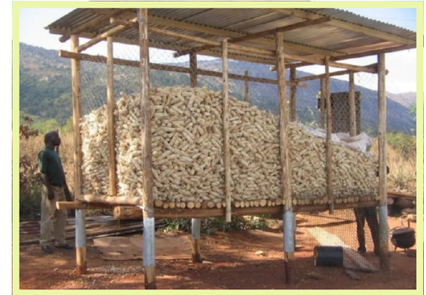
Figure 16: Good storage structure raised on poles with metal plates wrapped around the poles against rats
