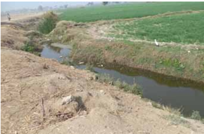
Figure 16: In Ghotki, a road borrow trench is serving as a local drain.
