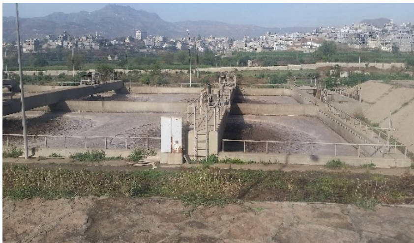
Figure 5: The wastewater treatment plant
